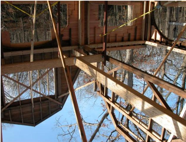
November 2004. Erecting the beams and supports in preparation of adding the second floor and the roof.
